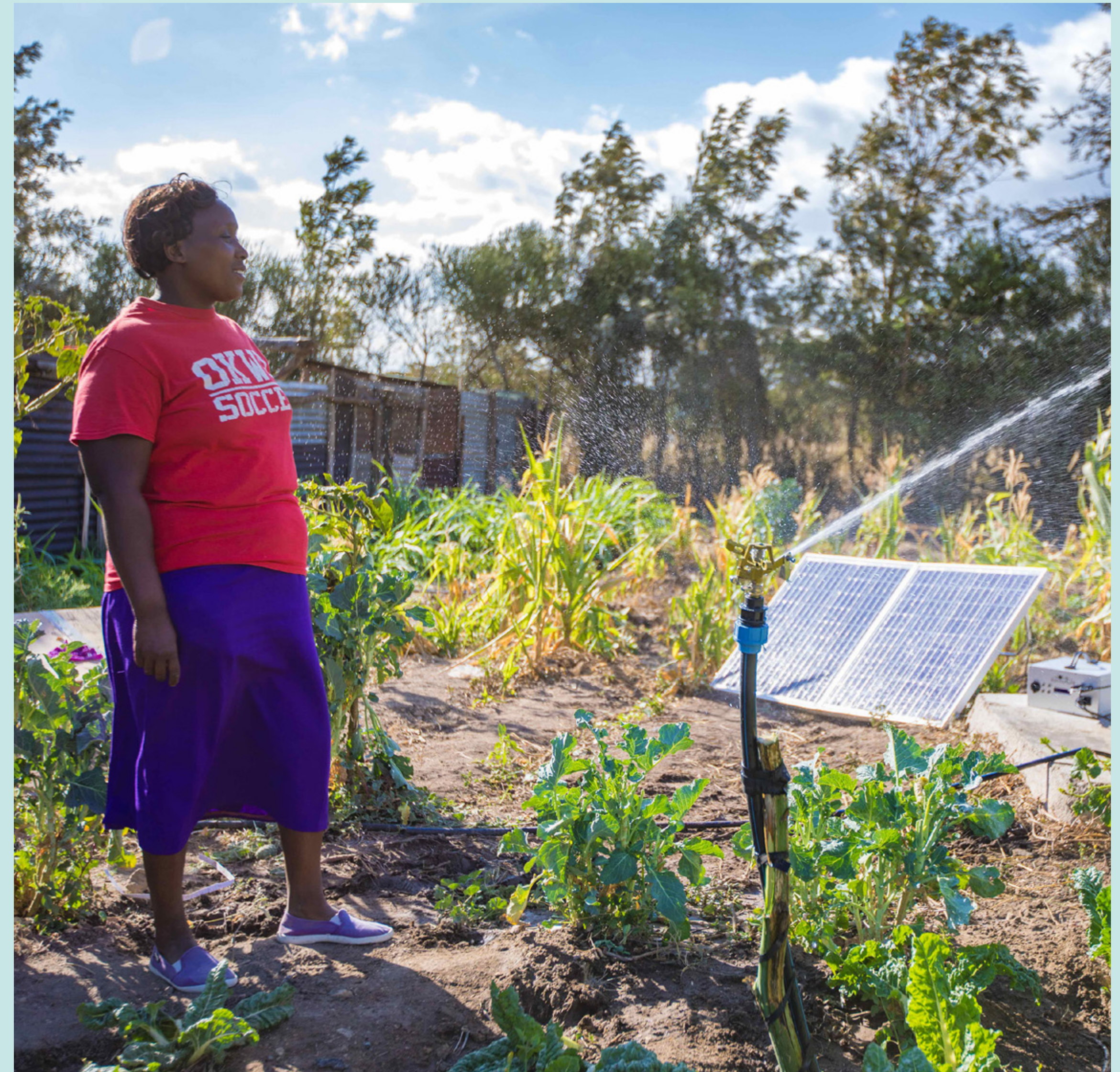
SunCulture provides a comprehensive offering, including solar water pumps. Photo: SunCulture.
